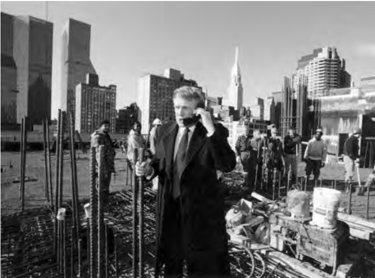
Donald J. Trump on top of Trump World Tower Construction.
