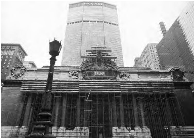
42nd Street Grand Central Station renovation.
